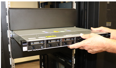
Figure 24. Installing the control enclosure
