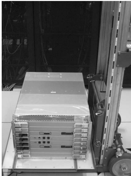
Figure 11. Lift tool and chassis positioned at rear of cabinet
