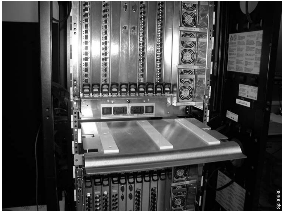
Figure 8. Locking the shelf into position
