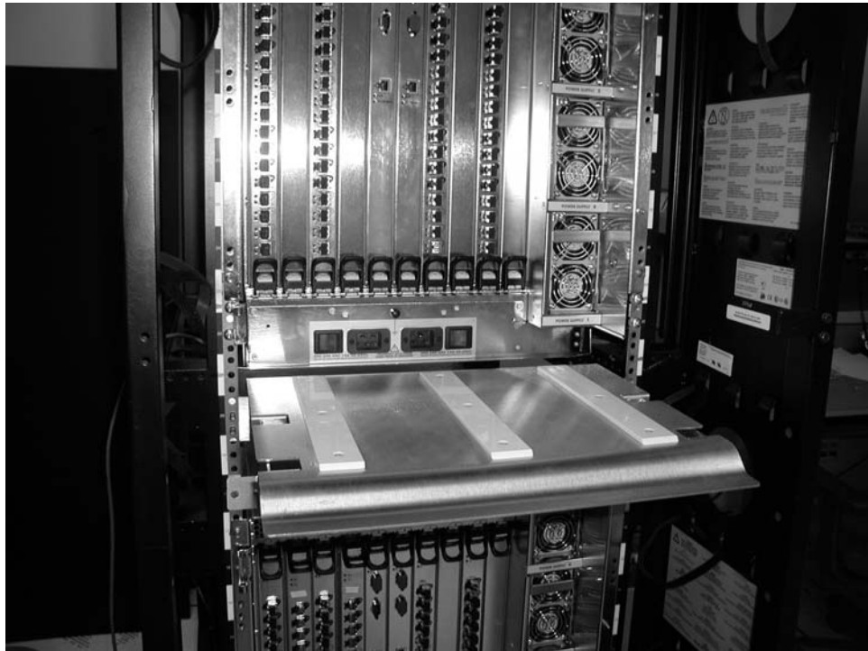
Figure 7. Locking the shelf into position
