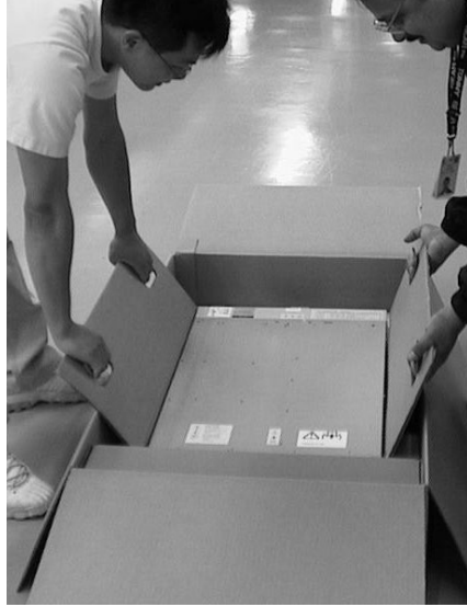
Figure 117. Two persons unboxing the uninterruptible power supply
